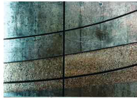
Precast concrete panels with incised lines/ varying finish
